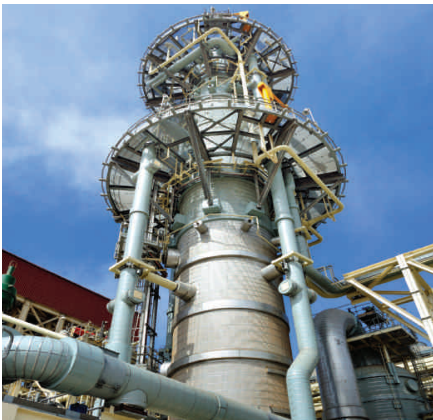
Bergen Pipe Supports range of hangers and cryogenic pipe supports used at a major LNG liquefaction plant in South America.
