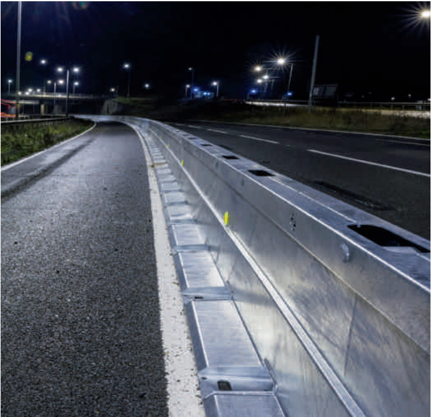
Zoneguard barrier installation on the A14, Kettering.
